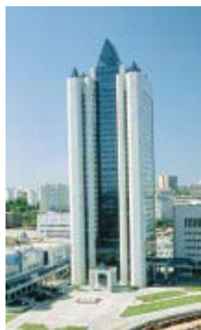
Gazprom Building, Moscow, Russia
