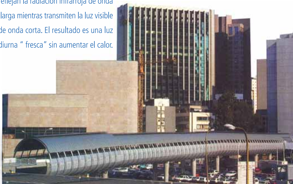
Walkway over Ayalon Freeway, Tel-aviv (Israel). Arquitectos: A.M.A.B. DP16 reflectivo 5800m 2
